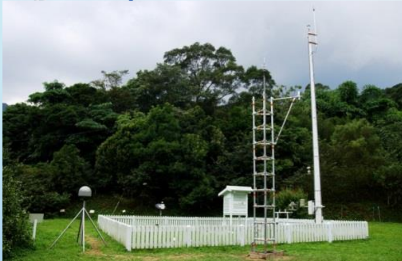
Hwa-lin Meteorological Station
